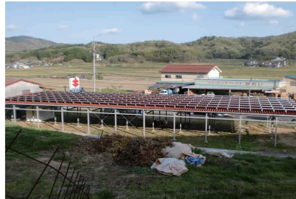
Tin Roof System(L feet)
